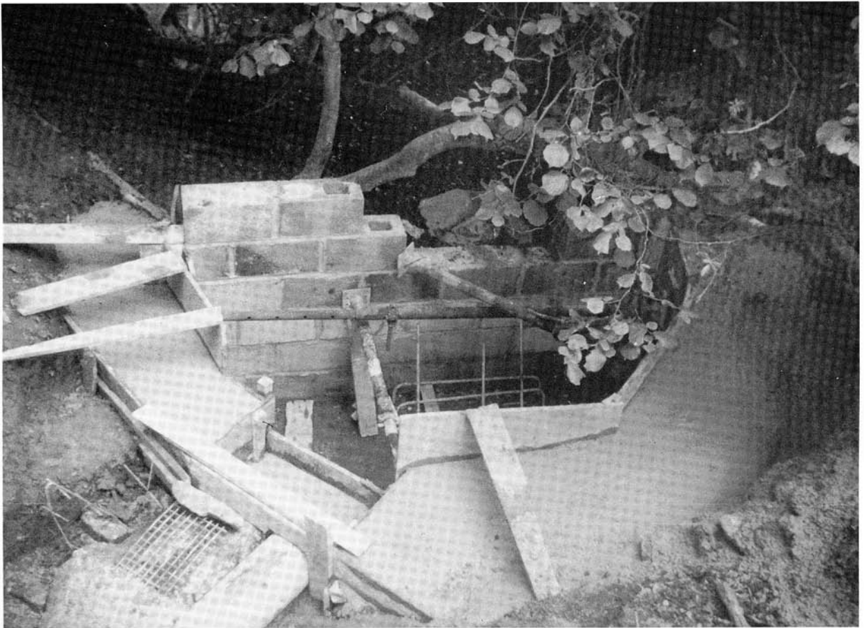
The settling tank upstream of the hole.
